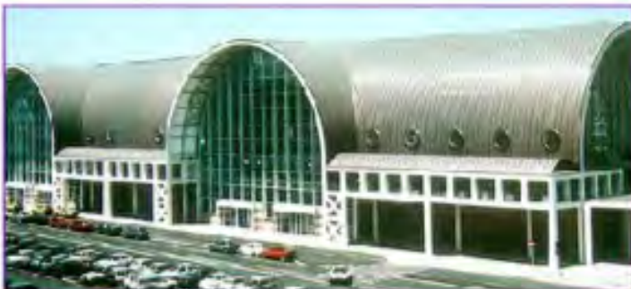
AIR TERMINAL Ostiense
